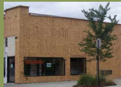
New facade in progress at the El Rancho building
