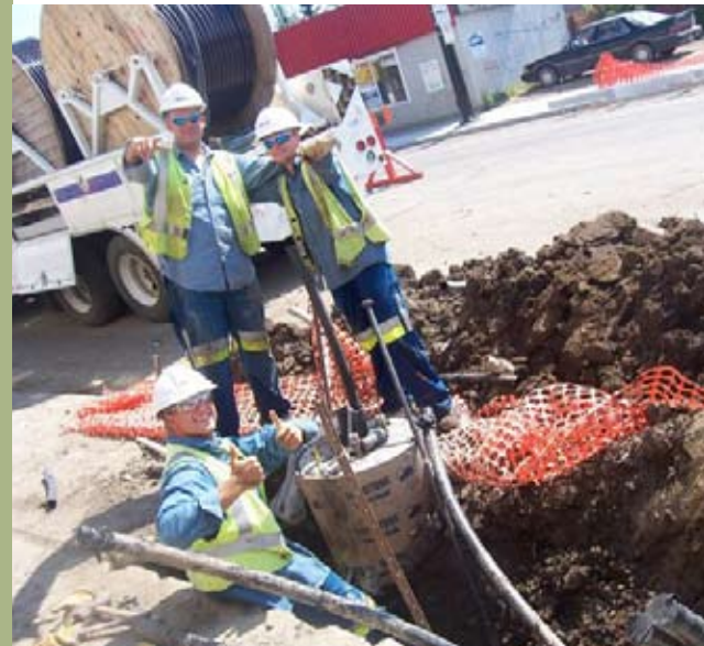
Construction workers on the job
